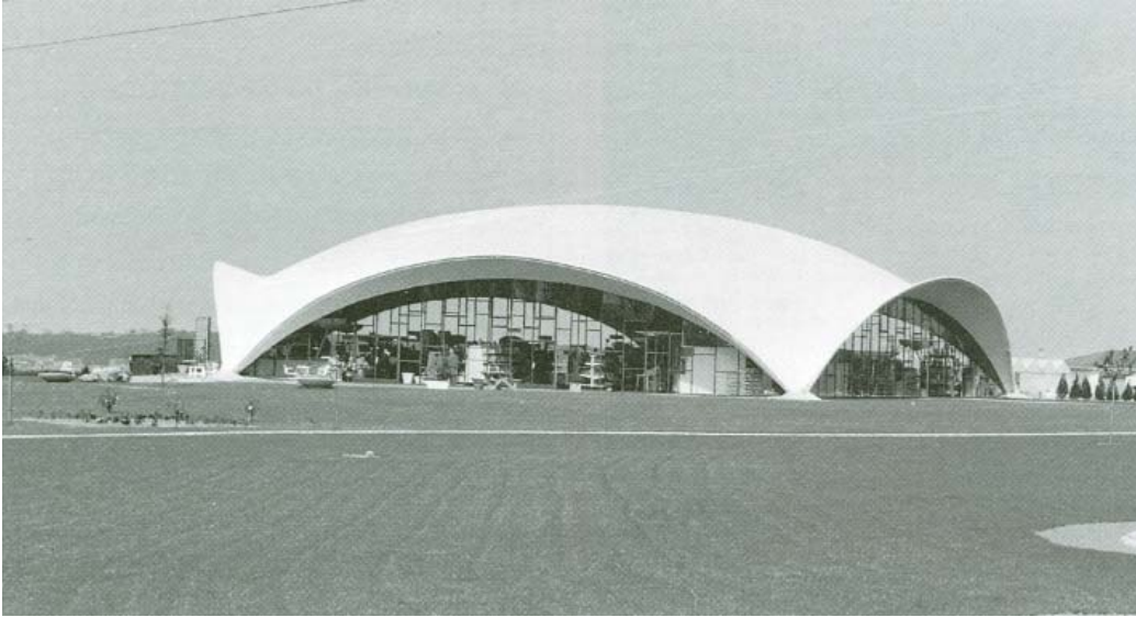
Figure 2. This garden center near Paris epitomizes the tendency for shell buildings to be designed as objects in a flat, empty field. Photo: Chilton, p. 81.
